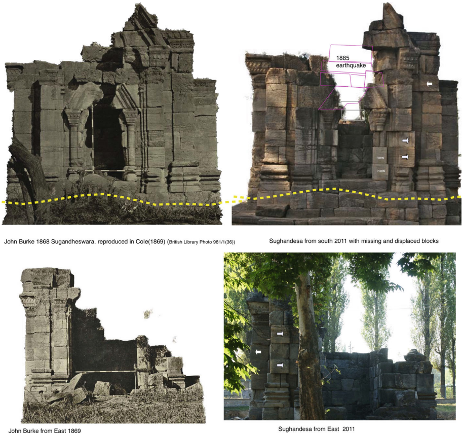
Fig. 13 Views of Sugandhesa: top pair from the south in 1868 (Cole 1869, left) and 2011 (right), and lower pair from the east, showing damage sustained in the 1885 earthquake, and evidence of toppled blocks that we interpret to have fallen in previous earthquakes. Arrows highlight lateral block motions typical of earthquake jostling. The gradation of the poles visible in the left hand figures are in feet
