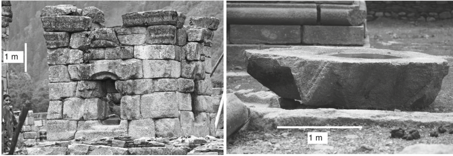
Fig. 9 The upper temple at Naranag and part of its granite roof lies inverted nearby. The monolithic roof measures 2.5 \times 2.5 \times 0.7 \text{ m}^3 . Note the absence of a masonry arch, and the assembly of walls from blocks of various dimensions
