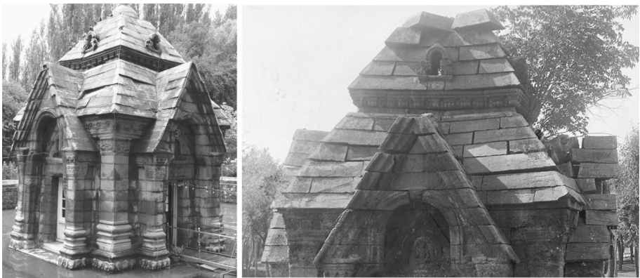
Fig. 7 The Pandrethan temple in 2006 (repaired in the twentieth century), with a close-up of the roof taken in 1903 after the 1885 earthquake. An earlier photograph in 1868 shows an identical misalignment of roof blocks ( Bilham et al. 2010 ) indicating that earthquakes before 1885 were responsible for the observed displacements
